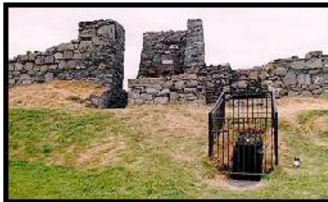
*The entrance to the Postern Gate (surrounded by the railings). In the thickness of the wall, directly above the entrance, is the "murder hole". To the left is a small tower protecting the flankworks.*
