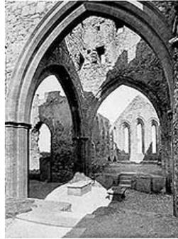
The *north transept* shows on its west face a small trefoil window, restored; its north gable end which has more than once been altered, has a recent flattopped doorway with window above. At the northeast corner is a rectangular enclosure, which looks like the remains of an open air font or, a baptistery to the original church, only if it were such its position is unusual.
