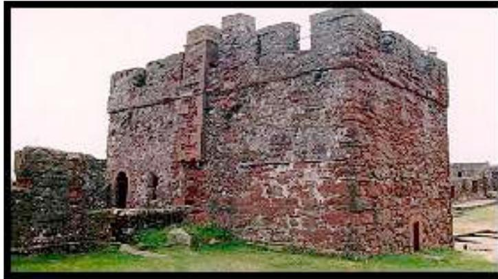
This is built of red sandstone with buff sandstone details. It consists of two storeys and a roof level with a fighting platform. The second storey is reached by a staircase within the thickness of the wall. In the 17th. century the second storey was the Constable's Quarters, as it was deemed the most suitable place for the tactical commander.
