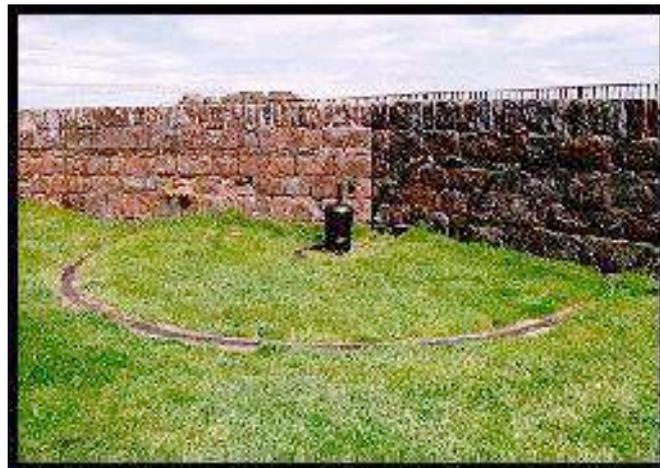
This is the site of the **New Battery**, built in 1816. An earth bank beyond the stone wall protected the guns. Old guns, buried upright in the ground, served as a pivot for the newer guns. The guns rotated on the metal track.
